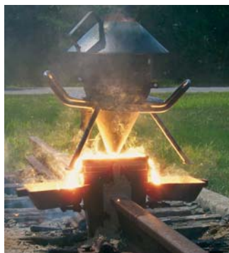
The molten iron formed in a thermite reaction is run down into a mold between the ends of two railroad rails. On cooling, the rails are welded together.
