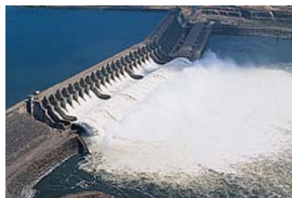
As the water falls over the dam, its potential energy is converted to kinetic energy. Use of this energy to generate electricity is called hydroelectric power.
