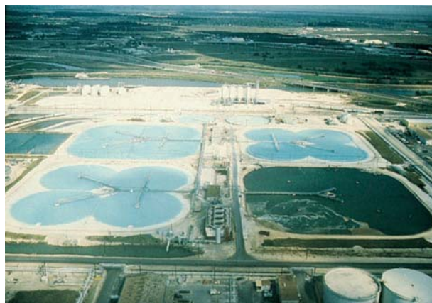
Magnesium hydroxide was precipitated from processed seawater in settling ponds at the Dow Chemical Company that once operated in Freeport, Texas.
