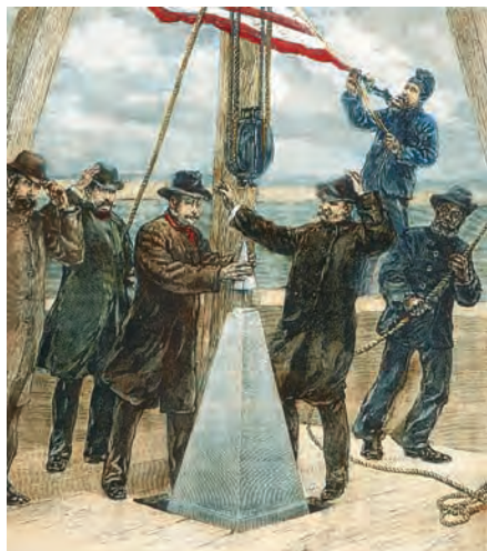
Setting the aluminum cap on the Washington Monument in 1884. At that time, aluminum was regarded as a precious metal.
