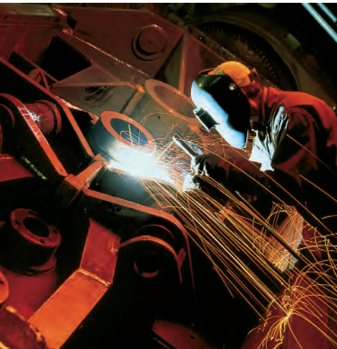
A worker using an oxyacetylene torch.
