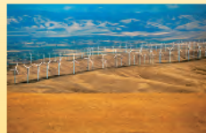
The State Line Wind Project along the Oregon-Washington border uses approximately 390 wind turbines to create enough electricity to power some 70,000 households.
