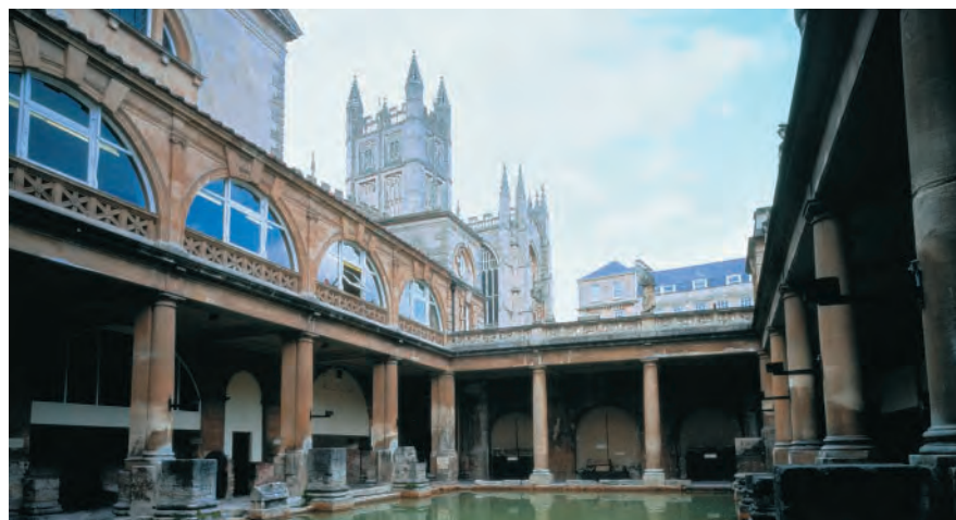
Roman baths such as these in Bath, England, used lead pipes for water.
